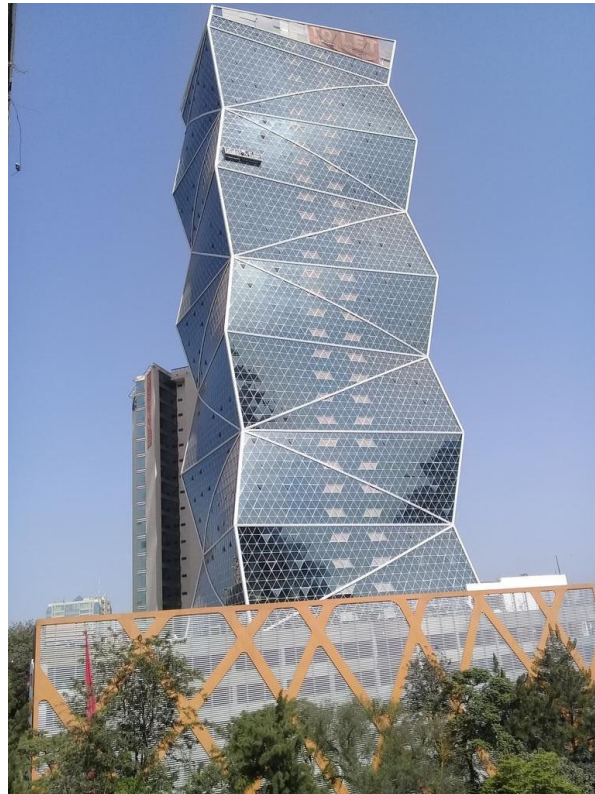
Kings Prism Tower, Upper Hill, Nairobi
